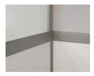
The ACT design creates a snug interior mounting of the insert panels, keeping them flush with the frame. This makes the assembled interior walls easy to keep clean.
