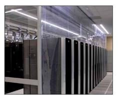
FlexSim<sup>™</sup> fire-rated curtains are the perfect choice for data center softwall containment.
