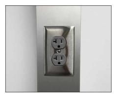
Flush mount, UL-listed 20 AMP / 120V electrical outlets are pre-wired in conduit that is concealed inside Simplex's standard wall panel framework.
