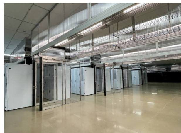
FIGURE 2 Ultima® AirAssure™ low leakage ceiling panels and DynaMax® structural grid.
